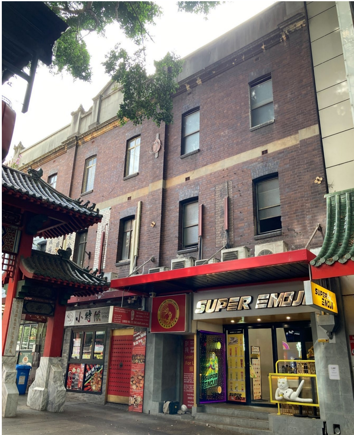
Figure 24. External view of 50-54 Dixon Street. Source: HAA, 2024.
