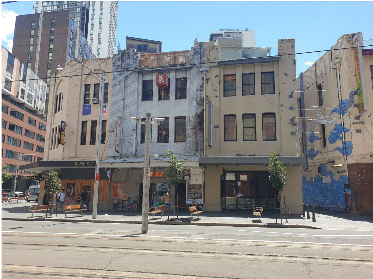
Figure 17 92 Hay Street, (centre building). Source Juanita Kwok, 2024.
