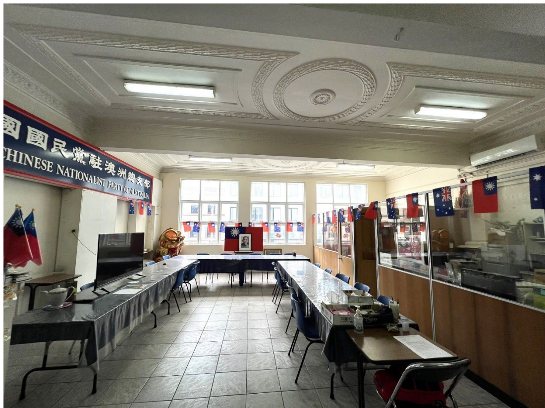
Figure 15 First floor office with plaster ceiling.
